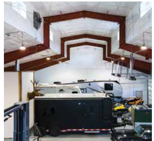
ENERGY SAVING SYSTEMS
